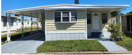
#4063 2BD/2BA This unit is a 1972, 660++sq ft. Updated 2026. There is plenty of natural light throughout the home. Open floor plan kitchen with a combined dining area. White kitchen cabinets with granite countertops. Stainless Steel appliances. Two new walk-in showers. This home offers a transferable roof over warranty for the lifetime of the home. Listed at $115,000
